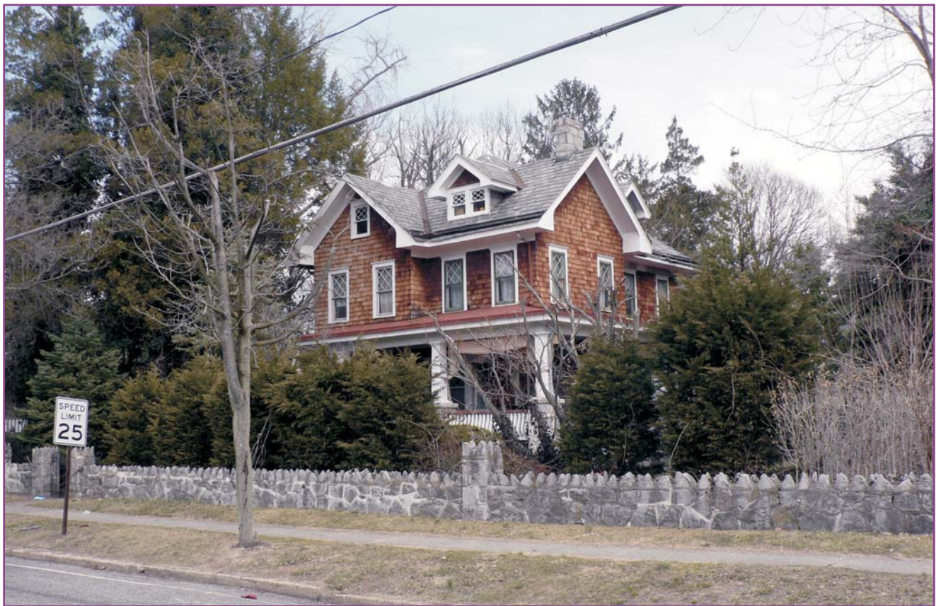
Photograph 1 of 46. View of 109 East Atlantic Avenue from the south showing the 2½ story shingled and sided frame building with slate roof and wrap around porch. Built circa 1913, the house is surrounded by overgrown vegetation that prevents full visibility.
