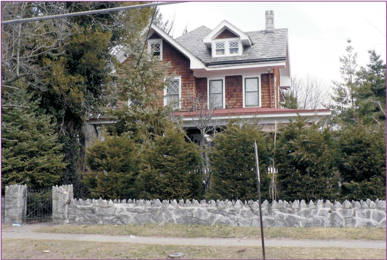
Photograph 2 of 46. View of the front (southwest) facade showing the stone garden wall with cast iron gate. The shrubbery directly behind the wall would have historically been pruned to match the wall's height.
